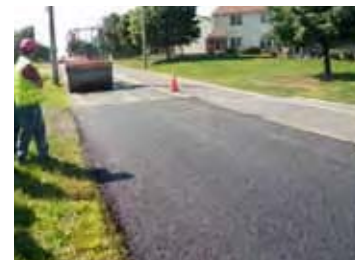
UTWC is placed in one lift with a final thickness of one to one and a half times the diameter of the coarsest or maximum-sized aggregate. (PennDOT photo)
