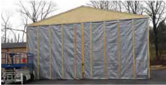
Salt shed entrance curtain, Whitehall Township.
