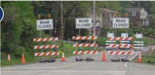
If you guessed photo 3, which shows a Road Closed sign on top of type III barricades, you are correct. MUTCD Section 6F.68 states: “Type III barricades should be used to close or partially close a road.”
